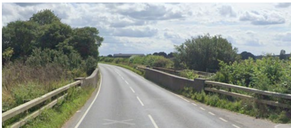
Figure 4.1 B430 / Chiltern Main Line railway bridge (image courtesy of Google)
