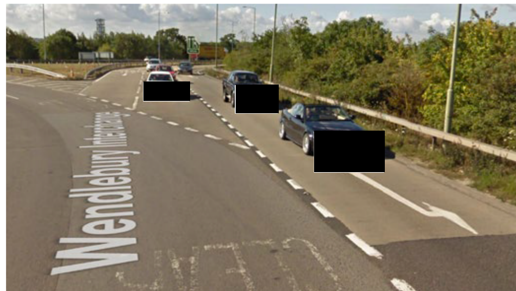
Figure 3.3 M40 Junction 9 A34 approach prior to 2010s scheme (image courtesy of Google)
